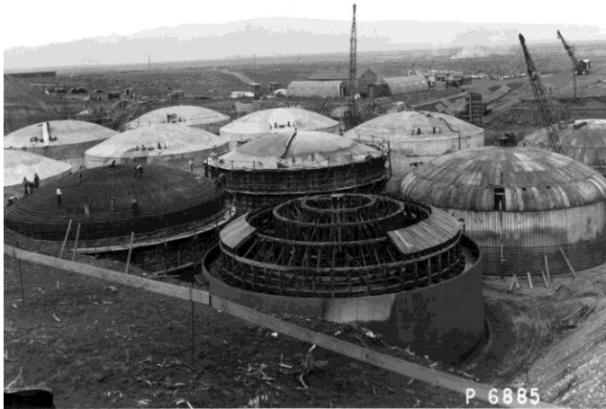
Single-shell tanks under construction in 1944 at Hanford
