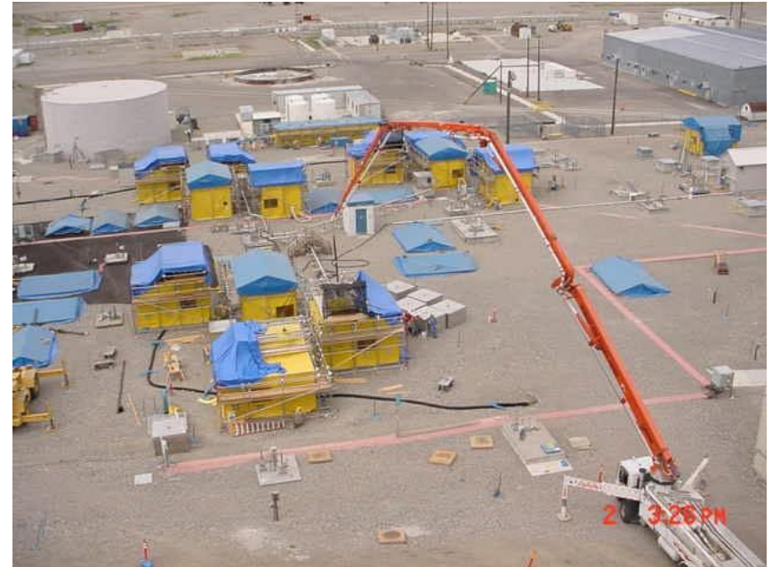
Tanks being Grouted
