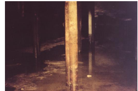
Supernatant in the tank NaOH liquor and most Cs-137
